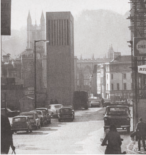
The first view of the Abbey at the time the book was written: a free-standing lift shaft-cum-fume extractor for the car park.
